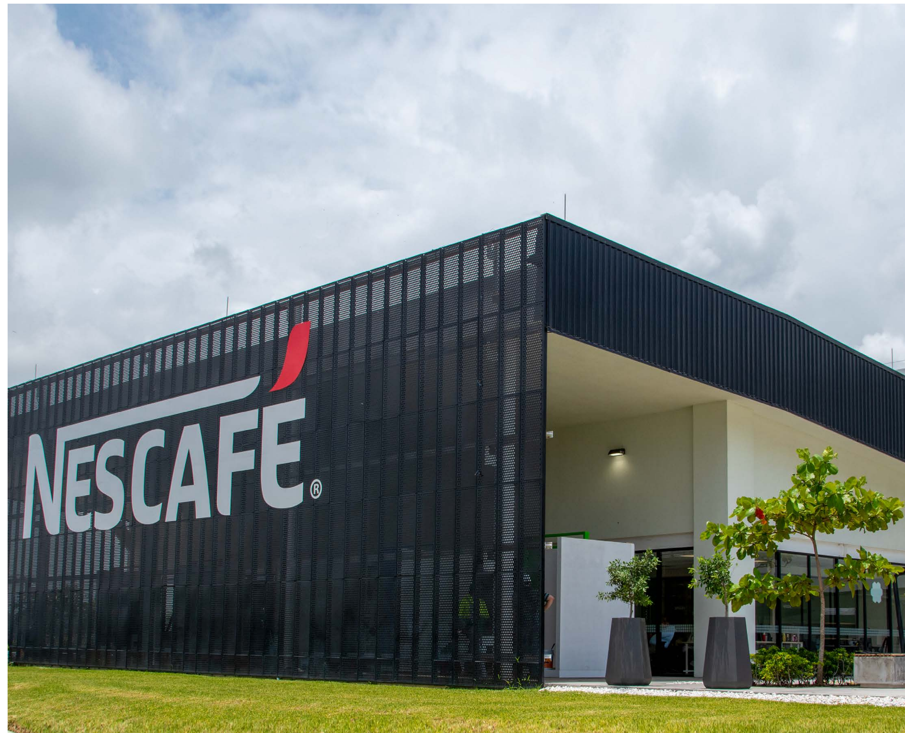
New Nescafé coffee factory in Veracruz uses state-of-the-art equipment to reduce water and energy consumption.
